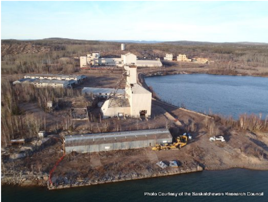
Figure 2. The Gunnar Mine Site Before Demolition of the Buildings in 2011.
