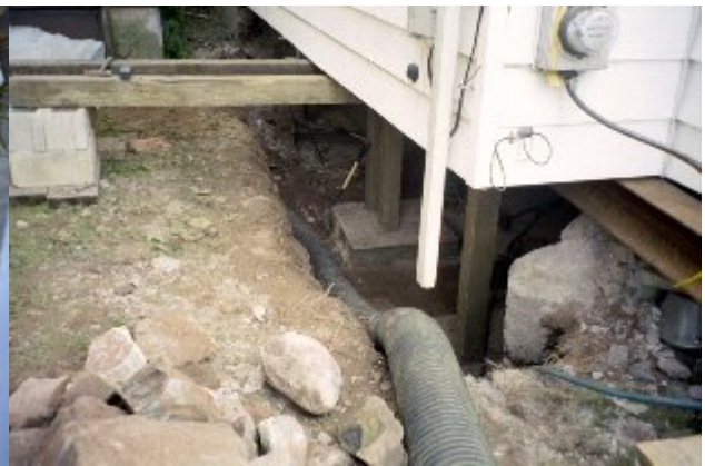
Fig. 5 – Field Stone Wall Removal
