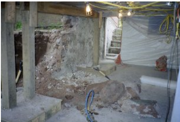
Fig. 4 – Field Stone Wall Removal
