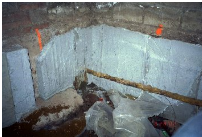
Fig. 3 – Foundation Underpinning
