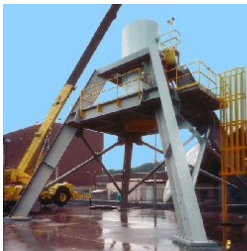
Figure 5 – Vertical Transfer using Shielded Transfer Cask System
