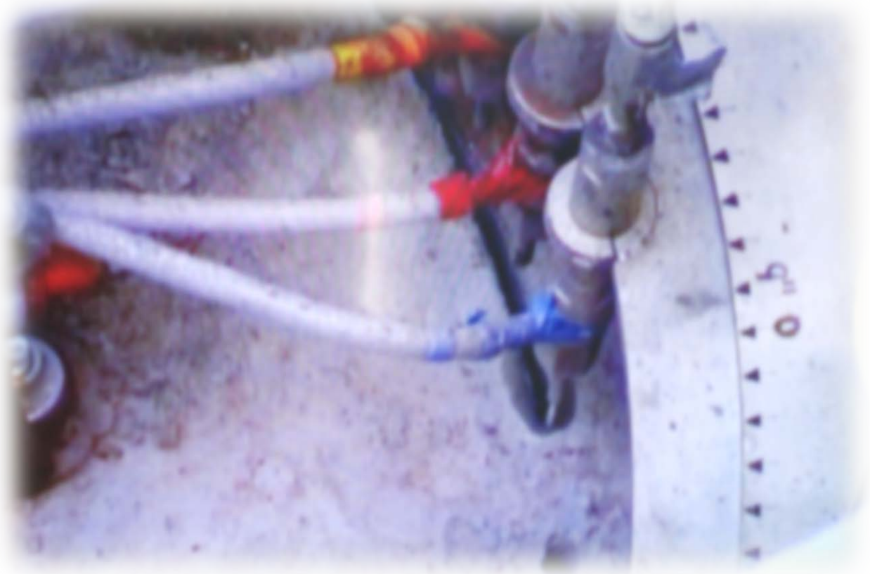
Fig. 4 - Single-Shell Tank Dome Cutting in Progress
