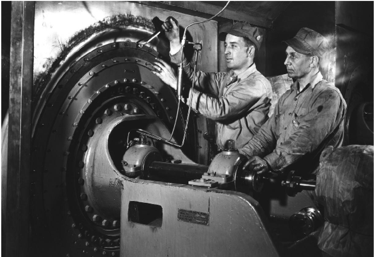
Figure 4. Workers performing maintenance on a cell housing in the K-25 uranium enrichment facility
