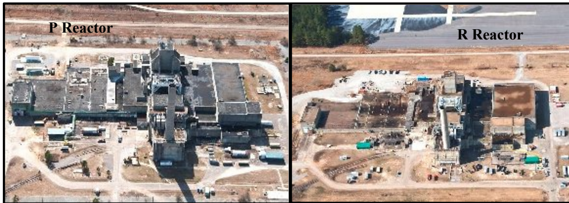
Figure 1 – SRS P and R Reactor Facilities before Decommissioning
