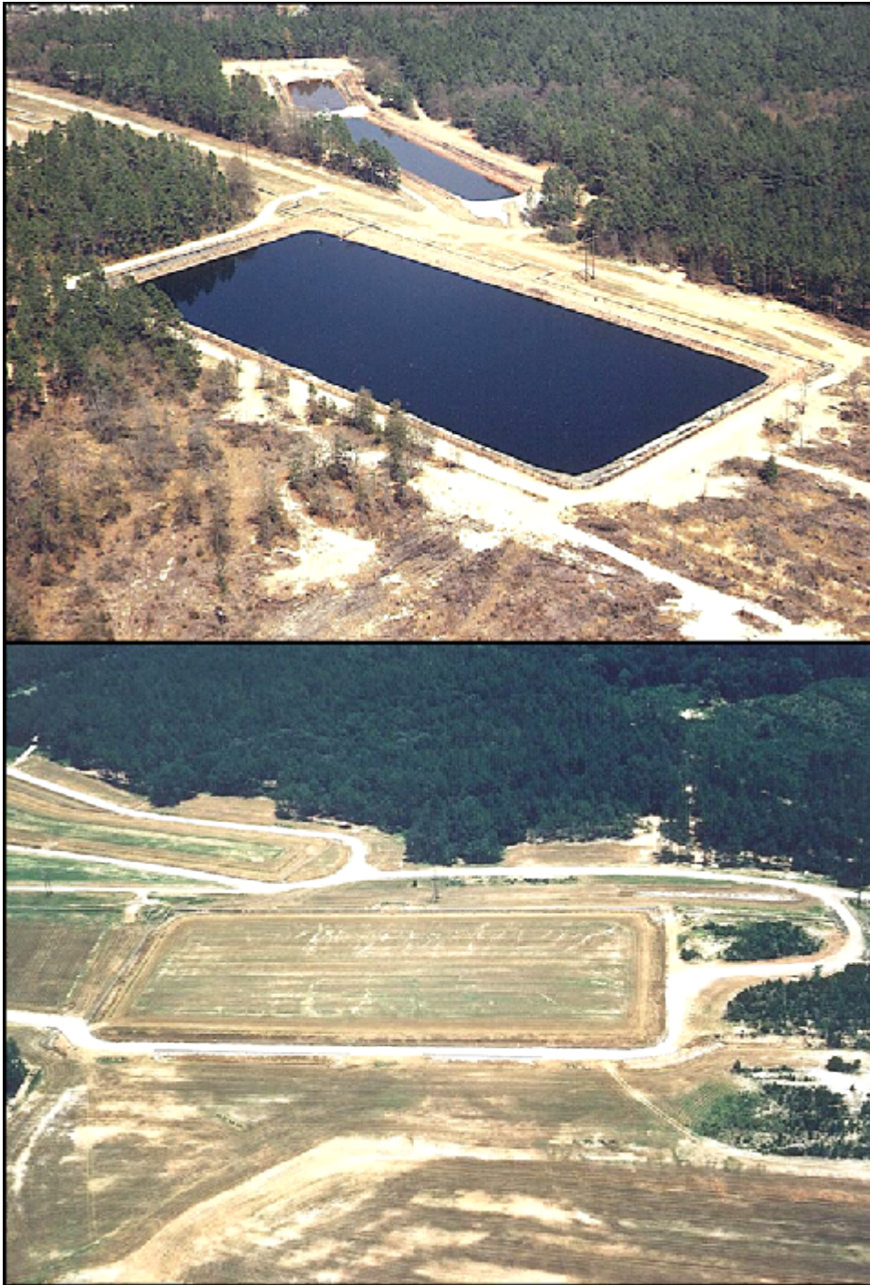
Figure 3. F Area Seepage Basins During Operations (top) and After Closure (bottom).
