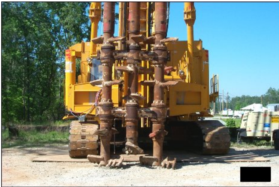
Figure 8. Soil Mixing Equipment Used to Construct the Groundwater Barriers.
