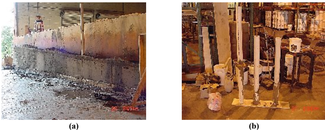
Figure 9. Final grout profiles and core samples. (a) T11-CC2 final profile and core sample. (b) Core samples from T10-CC1 long radius flow test.
