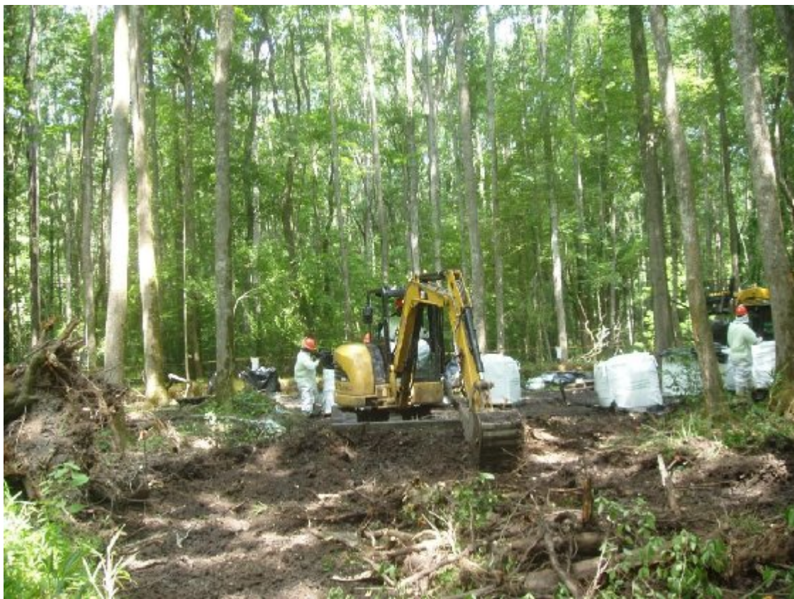
Figure 3. Removal Action of sediment/soil at Lower Three Runs
