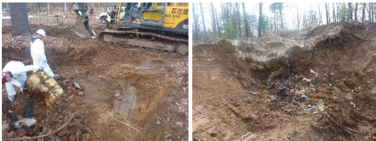
Photos 2 and 3. Excavation activities in the burial area.
