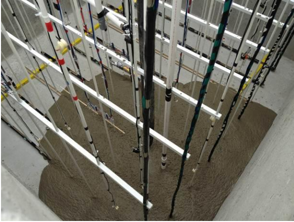
Figure 14. Grout Filling into Test Bed
