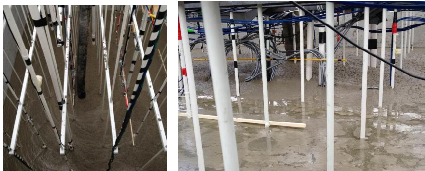
Figure 16. Grout Filling into Cube
