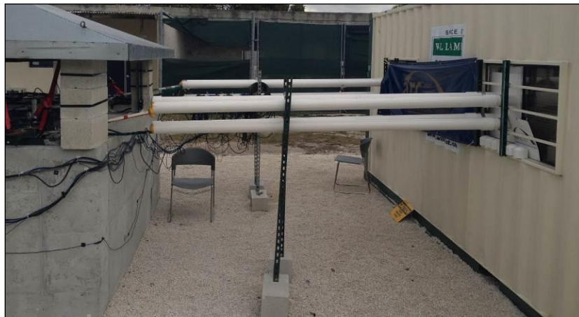
Figure 10. Cable routing system installed between test cube structure and office container.
