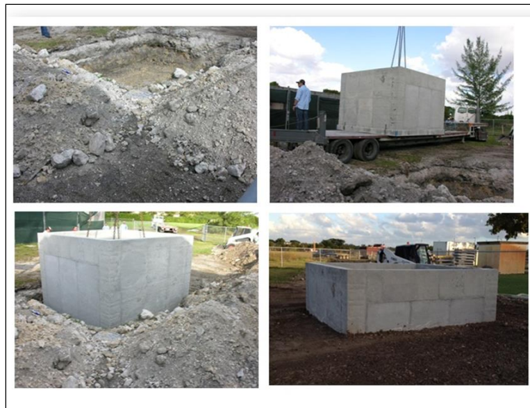
Figure 7. Installation of Cube
