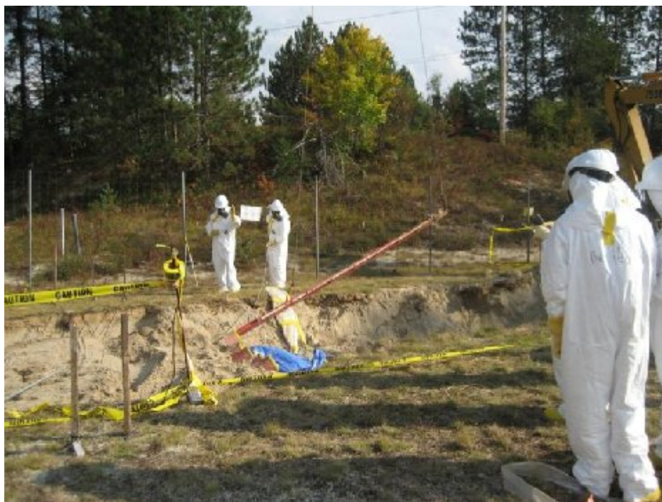
Fig. 6 Retrieval of the fuel rods and loading into new modern fuel cans with remote tooling and the angle iron.
