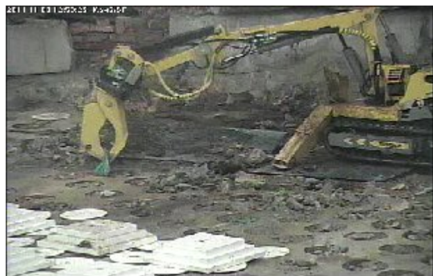
Figure 15 – Inside DSU 3B remote removal of debris using Brokk 90 robotic manipulator
