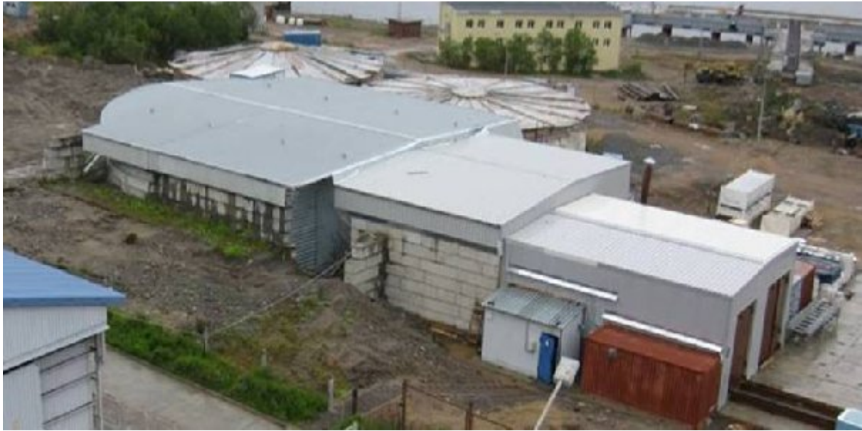
Figure 13 –DSU 3A with attached temporary process modules to carry out remote operations
