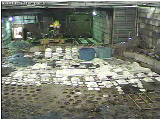
Figure 14 – Inside DSU 3B during installation of biological shielding
