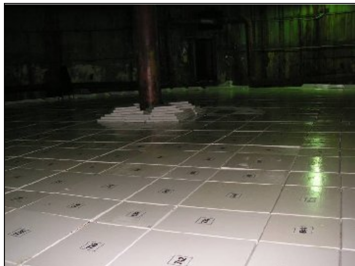
Figure 12 – Steel biological shielding greatly improved radiological conditions
