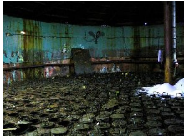
Figure 10 – Inside DSU 2B. Shield plugs were ill-fitting and snow could enter
