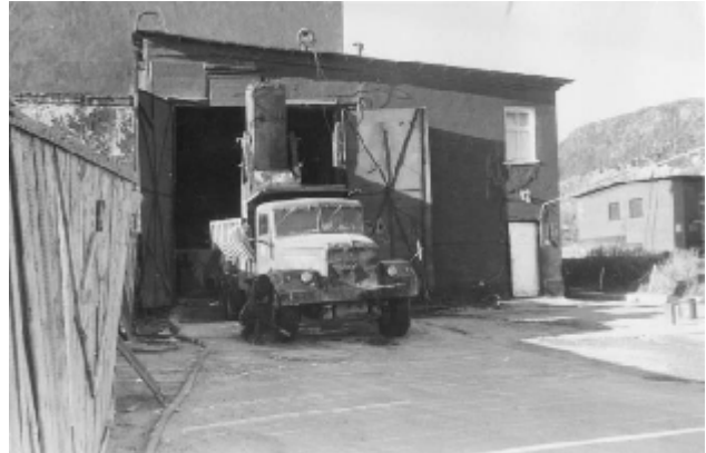
Figure 3 – Transferring SNF from the failed pond to the DSUs
