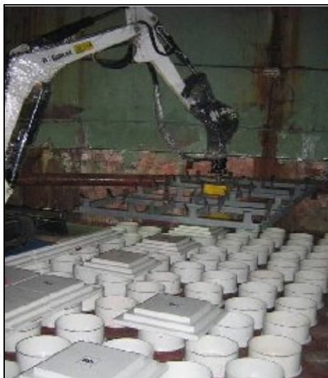
Figure 11 – Inside DSU 2B, Steel biological shielding was installed in 2010
