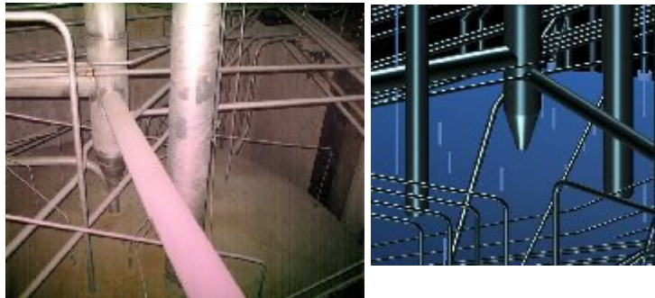
Fig. 9: A tank (left) and its 3D model (right), rebuilt by photogrammetry
