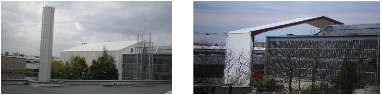
Fig. 6. Airlock in place over one third of the building
