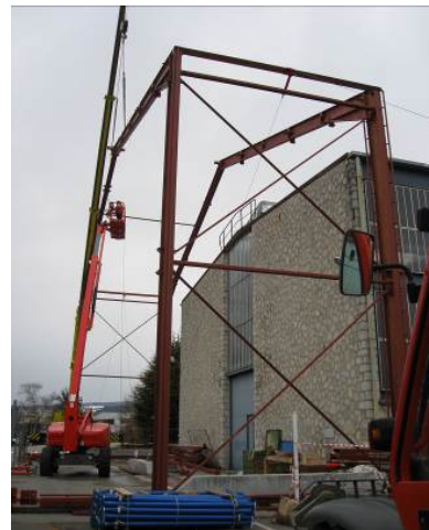
Fig. 5. Erection of the airlock
