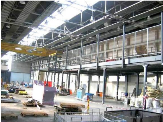
Fig. 7. Inside the building before the project
