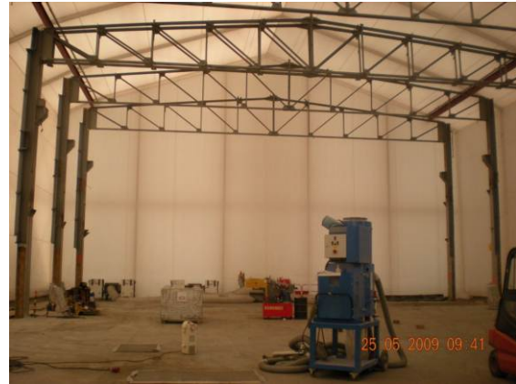
Fig. 8. Under the airlock after the demolition work
