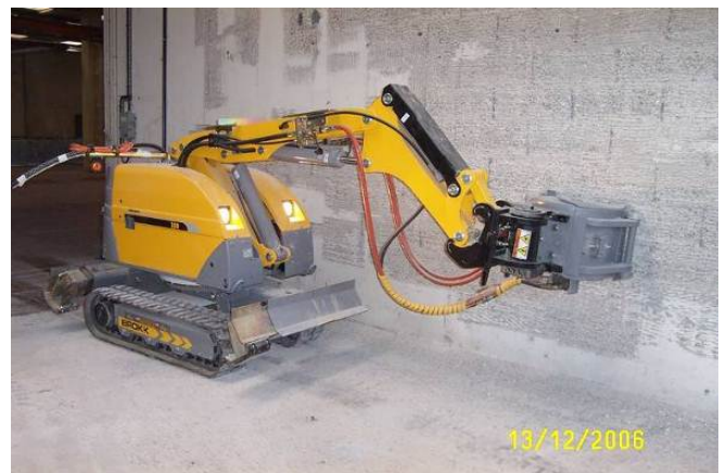
Fig. 3. Concrete scabbling using a Nuclearized Brokk
