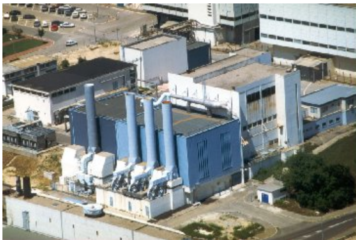
Fig.1: The vitrification facility
