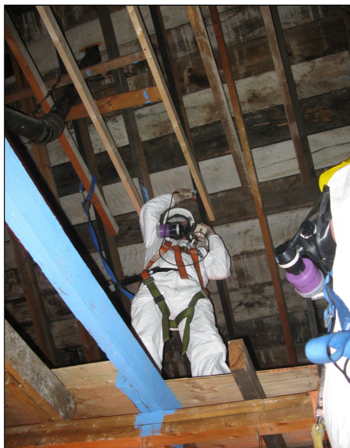
Fig. 6. Monitoring contact areas after removal of cross ties
