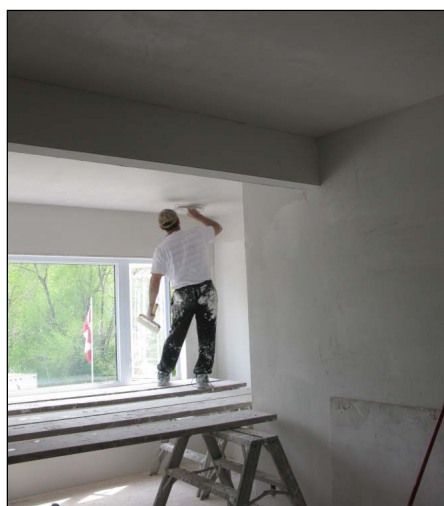
Fig. 7: Plaster work
