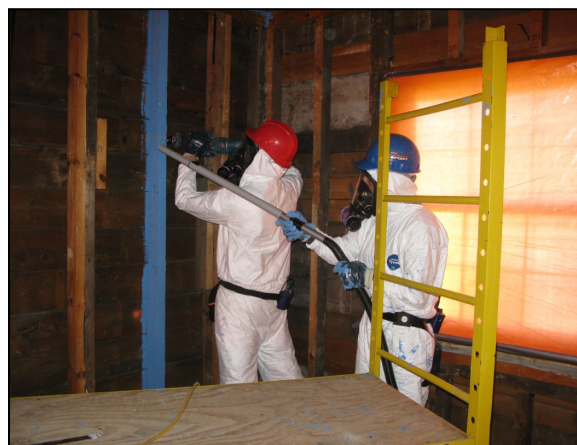
Fig. 3. Removing impacted stud (note HEPA vacuuming at cut)
