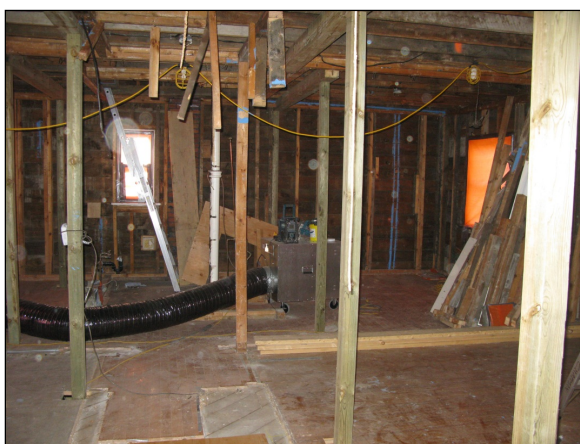
Fig. 4. Main floor with all walls removed (note HEPA depressurization unit)
