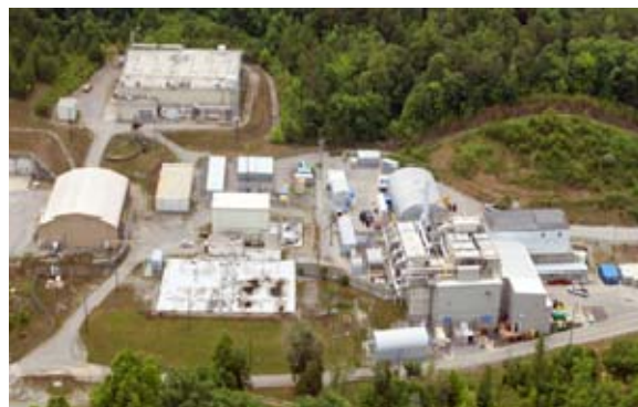
Figure 1 - TRU Waste Processing Center (TWPC)
