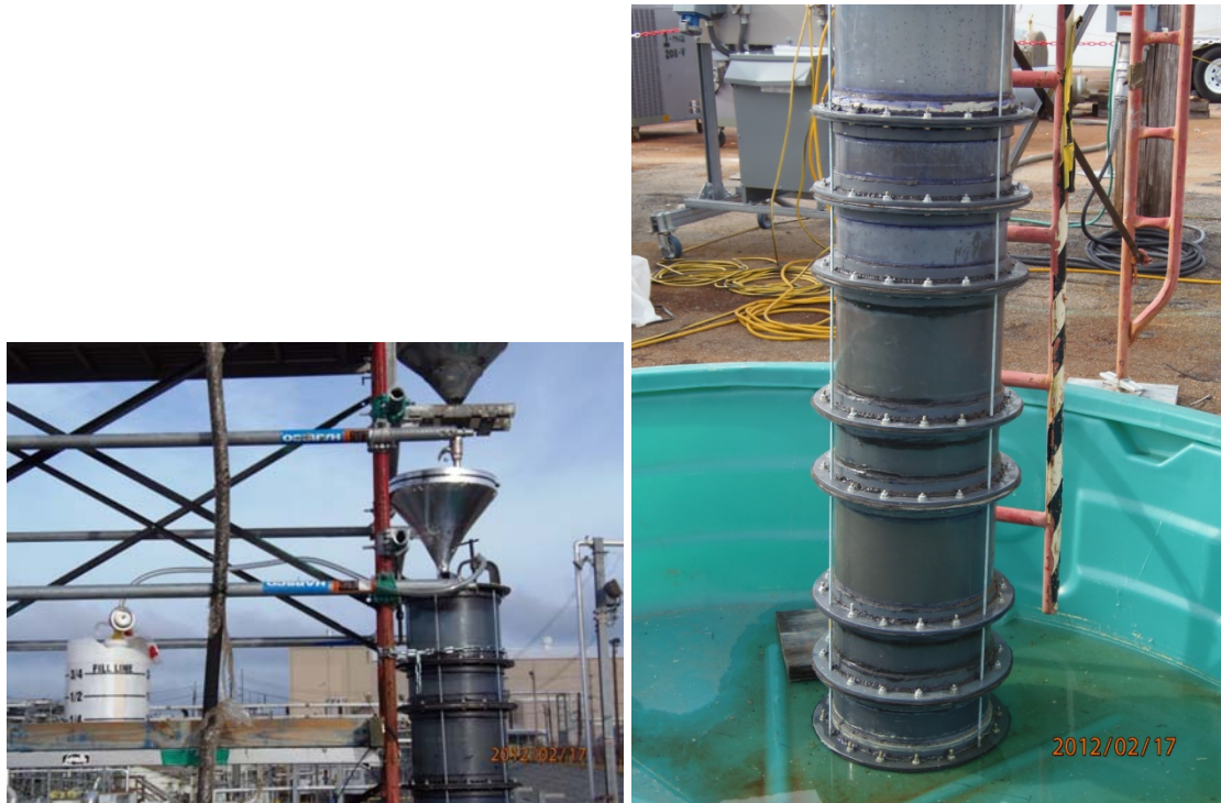
Figure 2. Equipment fill grout mock-up.
