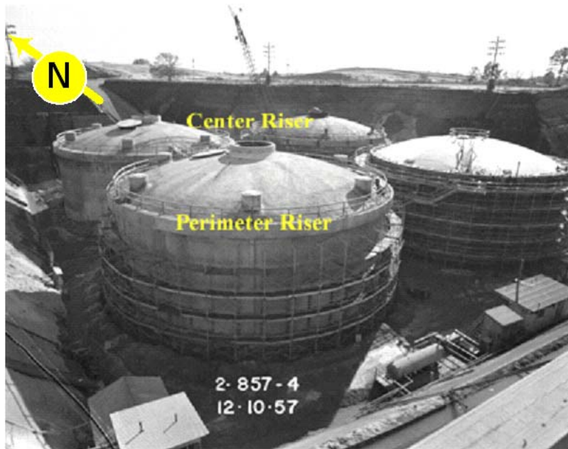
Figure 1. Tanks during construction
