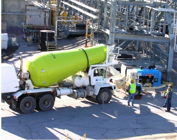
Figure 3. Grout Truck emptying bulk fill grout into Tank 19F
