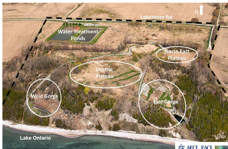
Fig. 1: Existing Port Granby WMF , [4]
