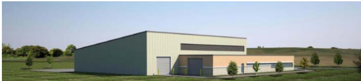
Fig. 6: Port Granby Waste Management Facility (WWTP), [4]
