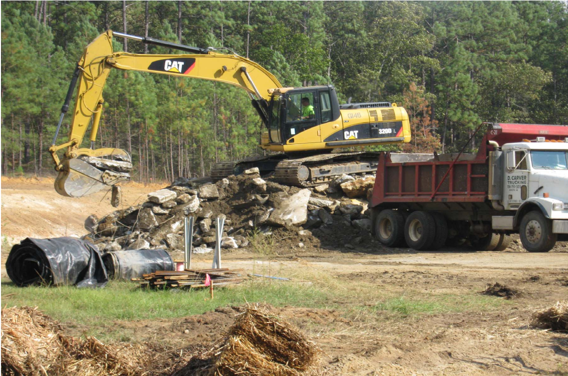
Figure 11. Loading of Concrete Debris into Dump Trucks at SATA
