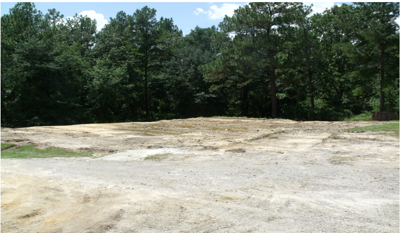
Figure 10. 661-G, Patrol Training Building, View Looking Northwest, After Demolition
