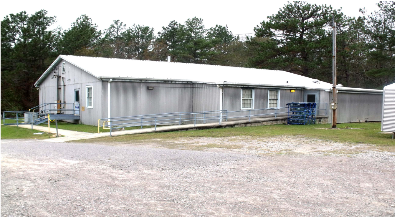
Figure 9. 661-G, Patrol Training Building, View Looking Northwest Before Demolition
