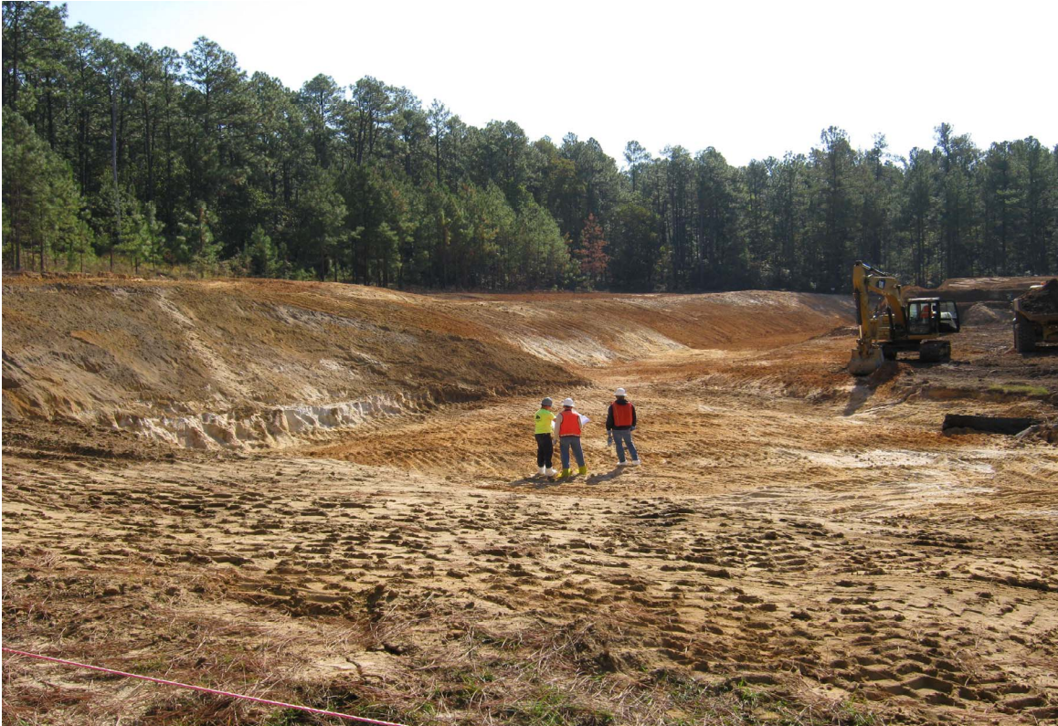
Figure 12. Removal of Lead and Lead Contaminated Soil
