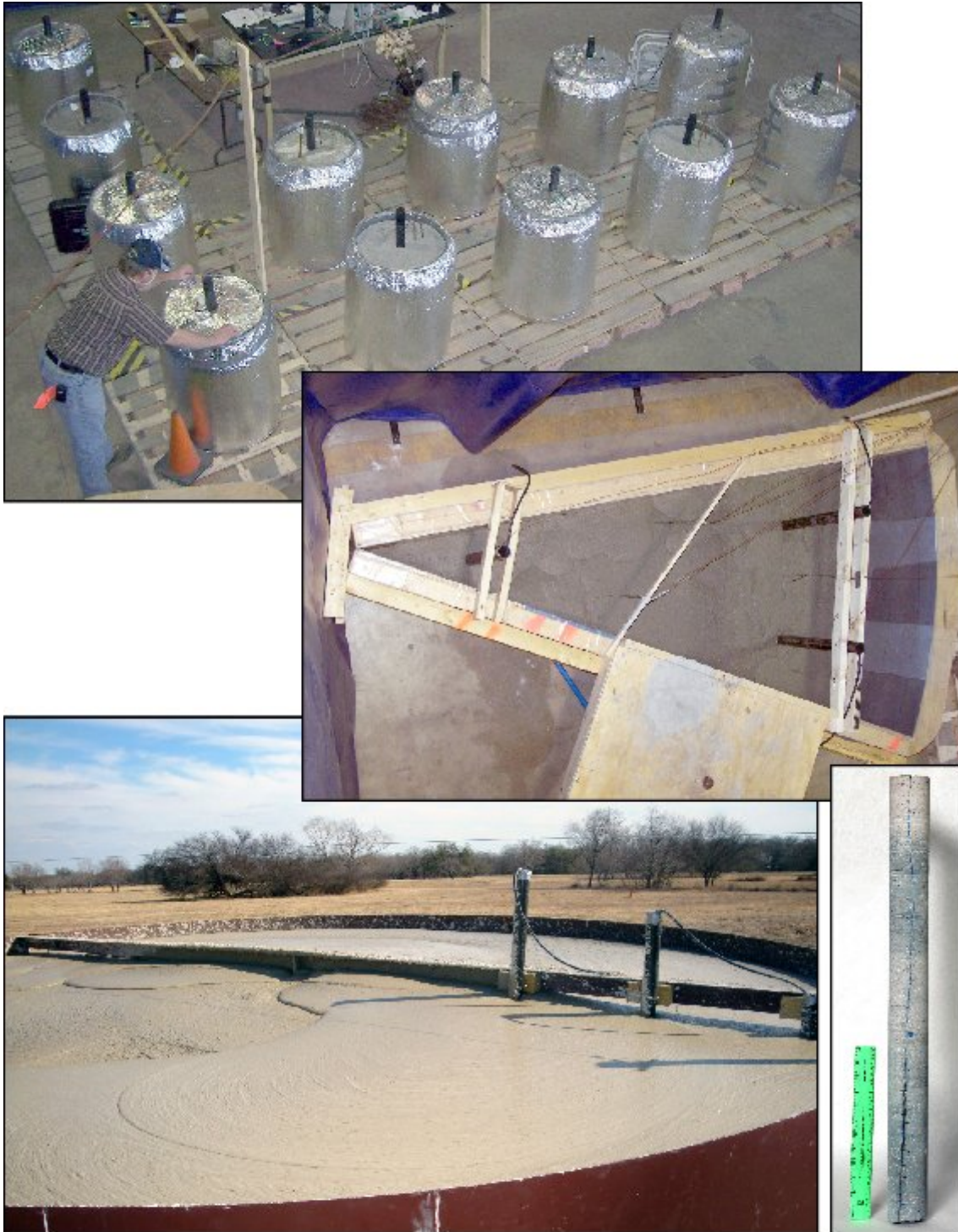
Fig. 1. (A) 55-gal drum-scale tank grout specimens. (B) Sector-shaped specimen, having 3-m radius by 30° arc by 0.8-m thickness. Pipes suspended in (A) and (B) were later filled with pipe grout. (C) Cylindrical specimen, 12× larger than sector, placed in a 0.63-cm-thick-walled tank, 6.1-m-diameter by 0.9-m-deep. (D) Cracked core extracted for analysis from (C).
