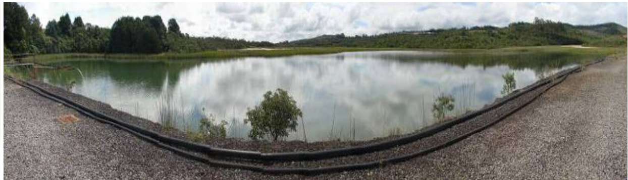
Figure 4 – The Tailings Dam
