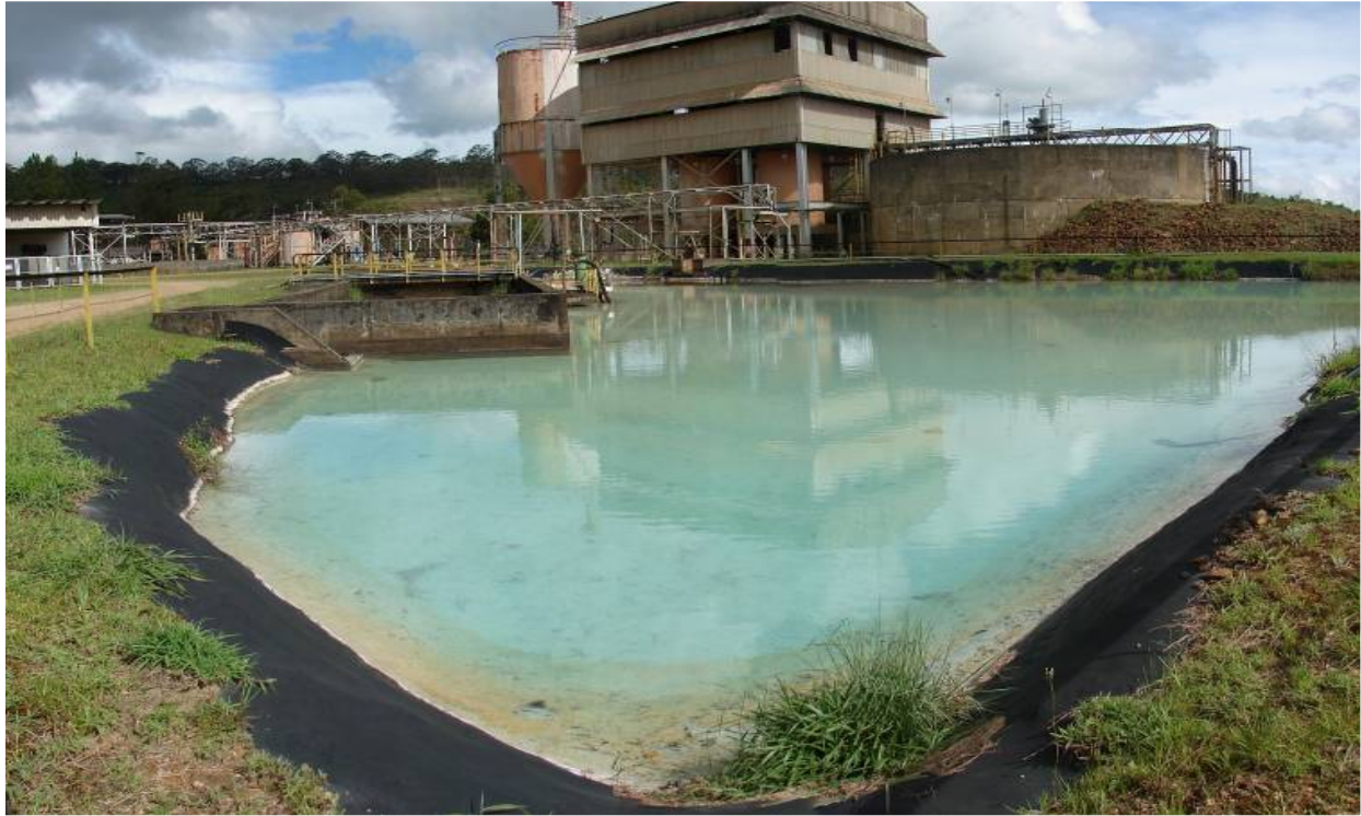
Figure 3 – Water Neutralisation Plant
