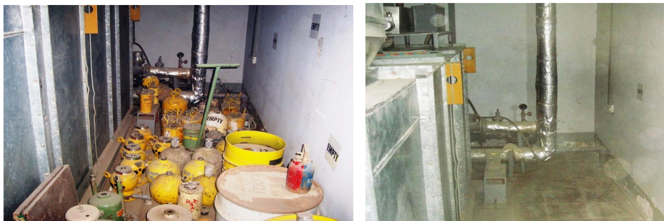
Figure 6. Before /After Photographs of one corner of DSRS Storage Bunker
