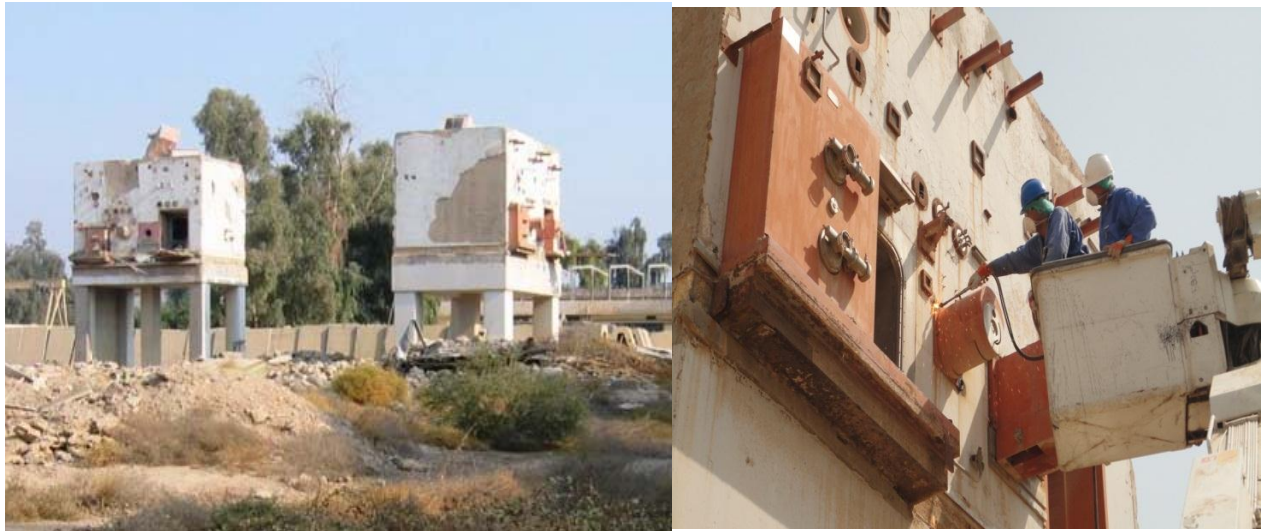
Figure 8. IRPL Hot Cells during Decommissioning
