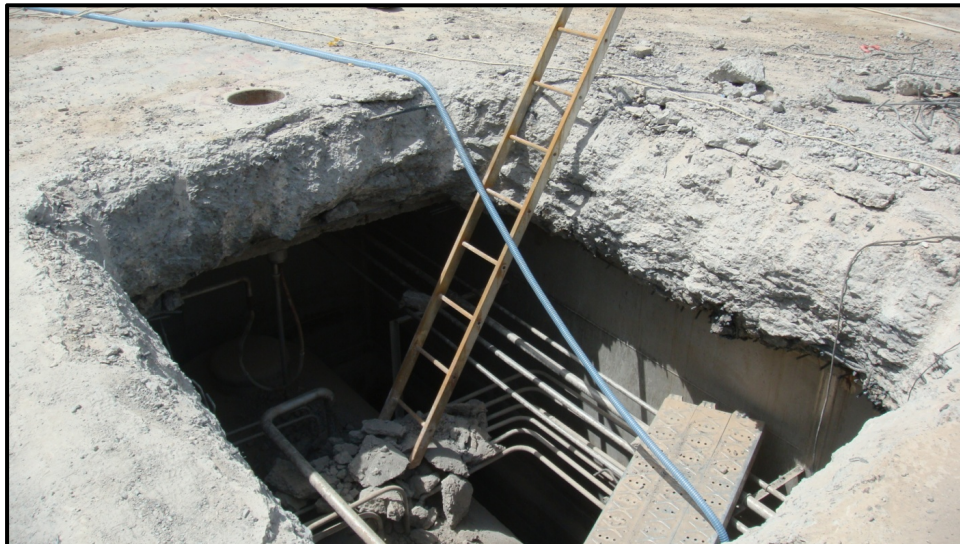
Figure 3. Recently Opened Radioactive Waste Tank Vault
