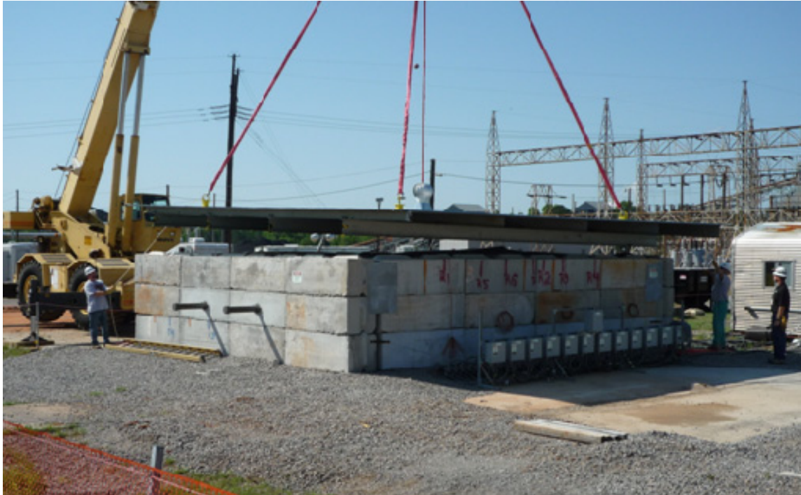
Figure 5: Final assembly of treatment cell used during the treatability study.
