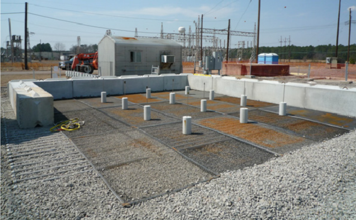
Figure 4: Initial assembly of treatment cell used during the treatability study.
