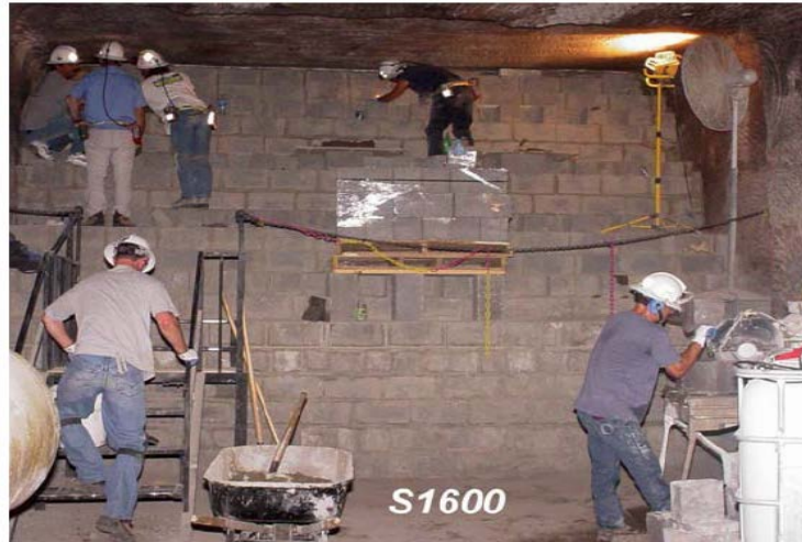
Fig. 3. Panel 1 block wall construction.
