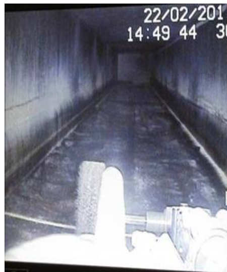
Fig. 10. Duct floor after brushing
