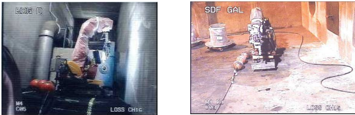
Fig. 9. MD duct cutting (left) and duct gallery vacuuming (right) using EDM
