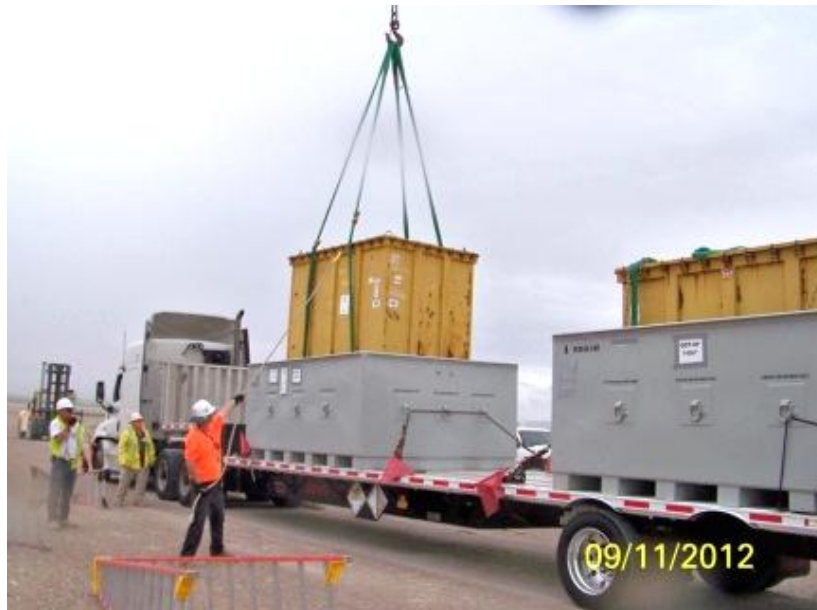
Fig. 8. Unloading the inner container for disposal at NNSS.
