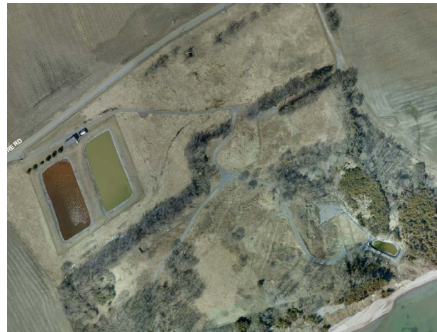
Figure 2 Port Granby waste management facility
