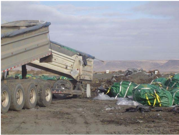
Figure 7 Off-loading - Grandview Idaho landfill
