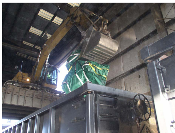
Figure 6 Unloading bags Mayfield, Idaho
