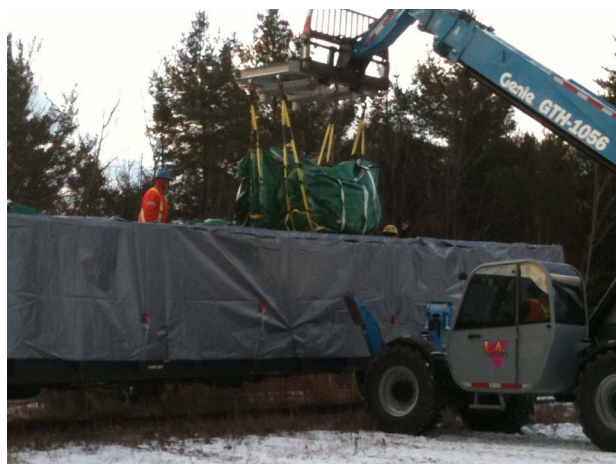
Figure 5 Off-loading at Rail Siding
