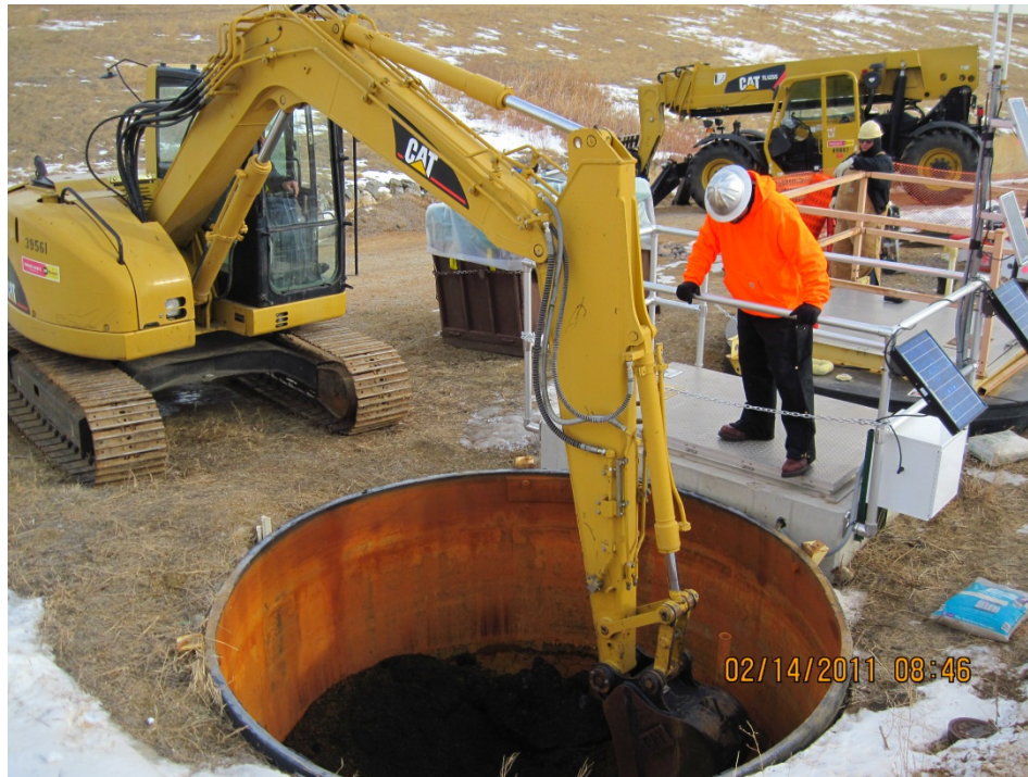
Figure 4. Removing spent MSPTS ZVI media.
