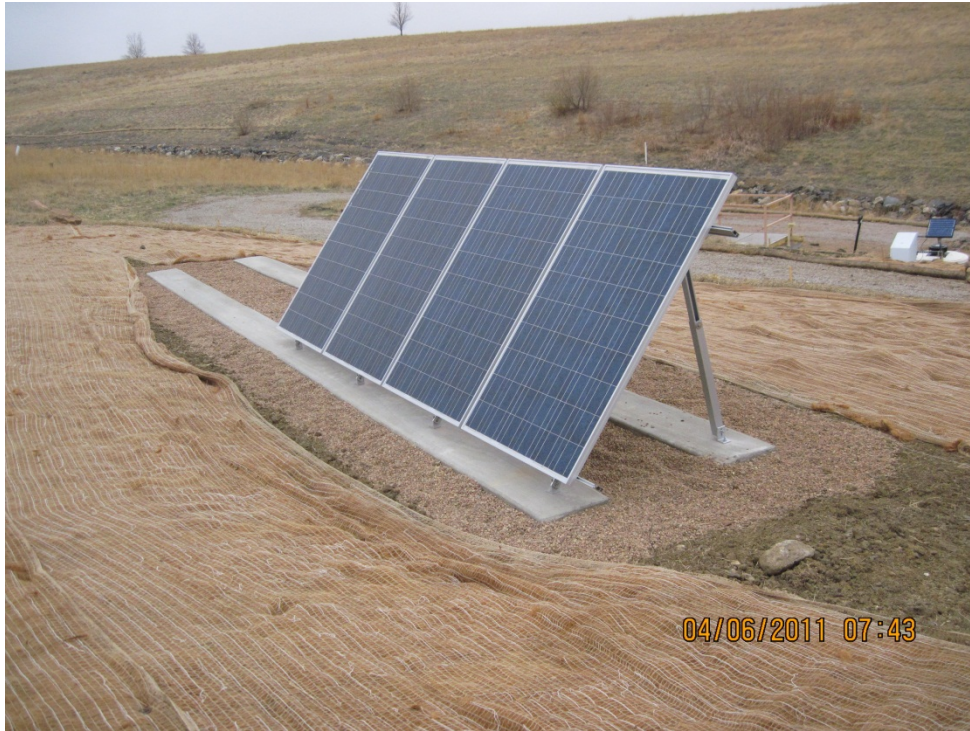
Figure 1. MSPTS PV array for air stripper.
