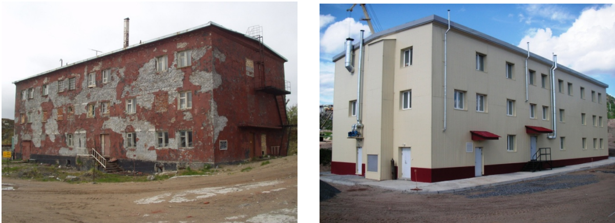
Figure 3. Radiation safety service building
