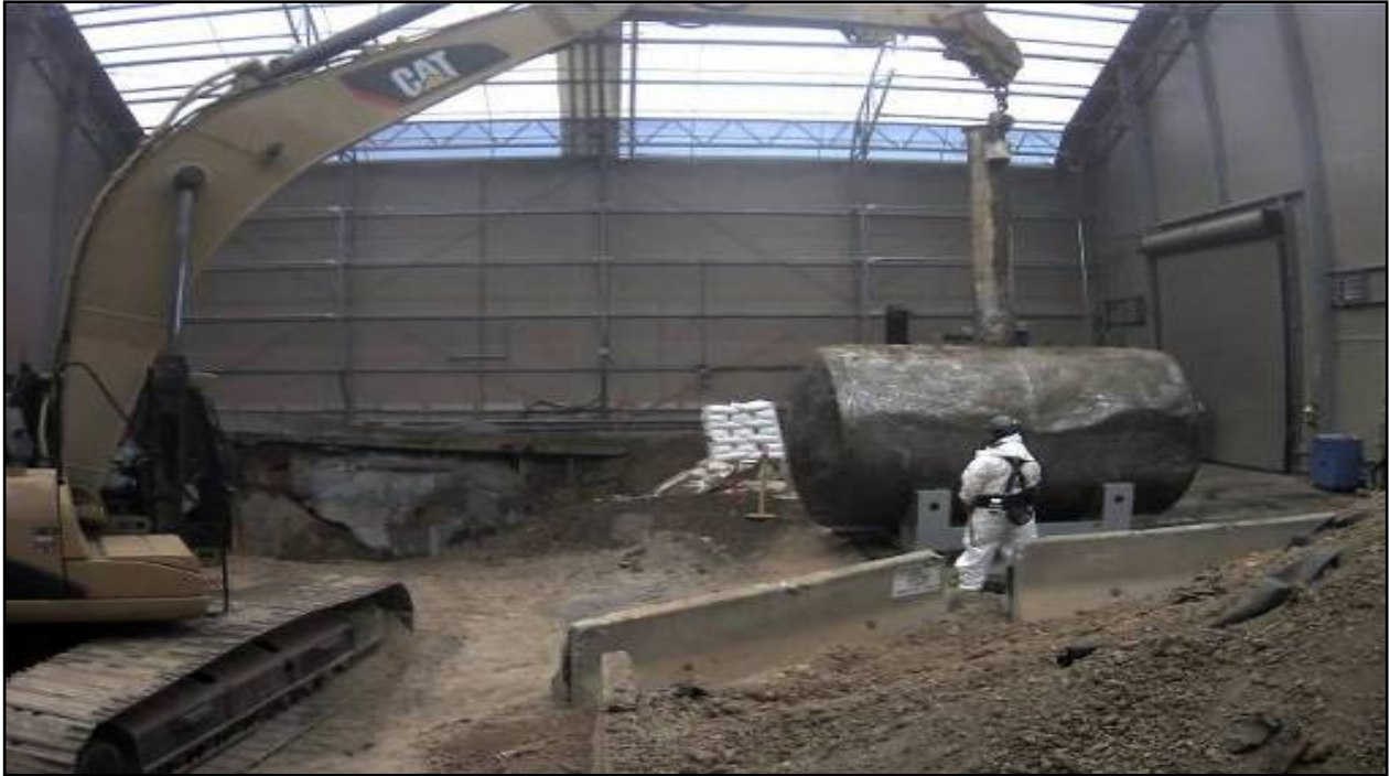
Figure 3. Removal of Tank W-1A
