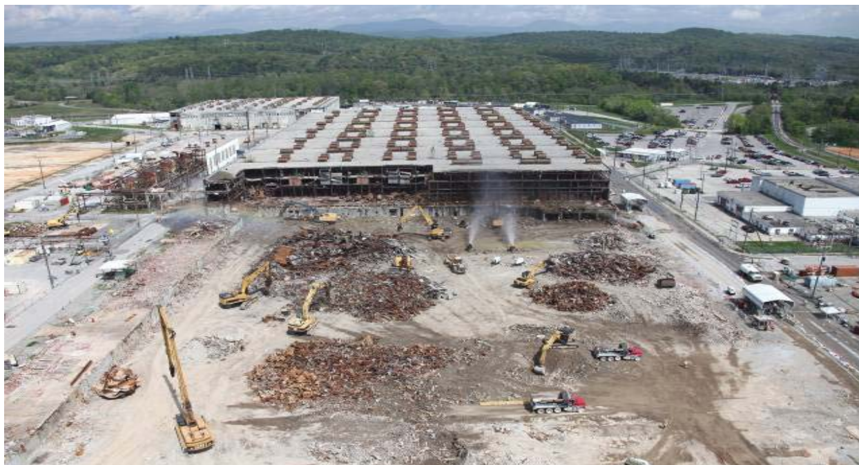
Figure 2. Demolition of the non-technetium-99 area of K-25's east wing
