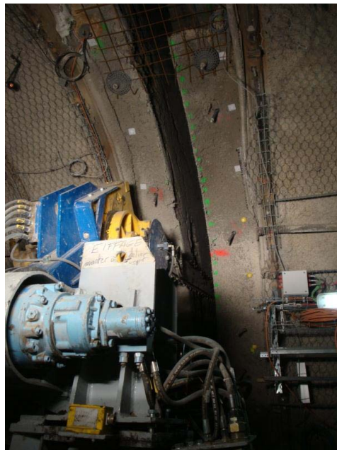
Fig. 4. The EDZ cut-off: groove sawing prior to backfilling with bentonite blocks.
