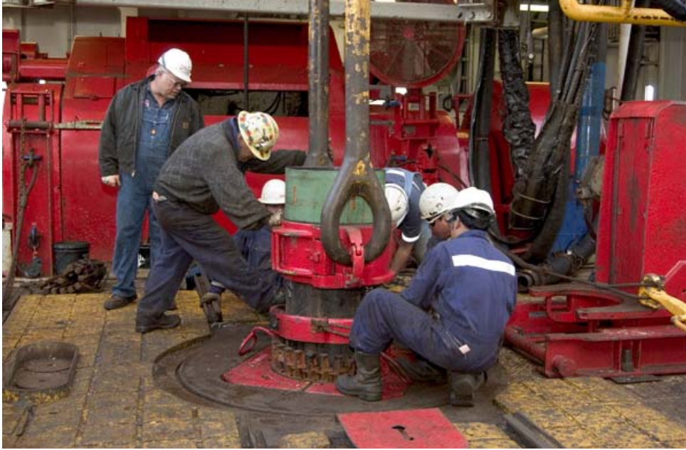
Fig. 4. Large Bore Casing in Rotary Table on Drill Floor [13].
