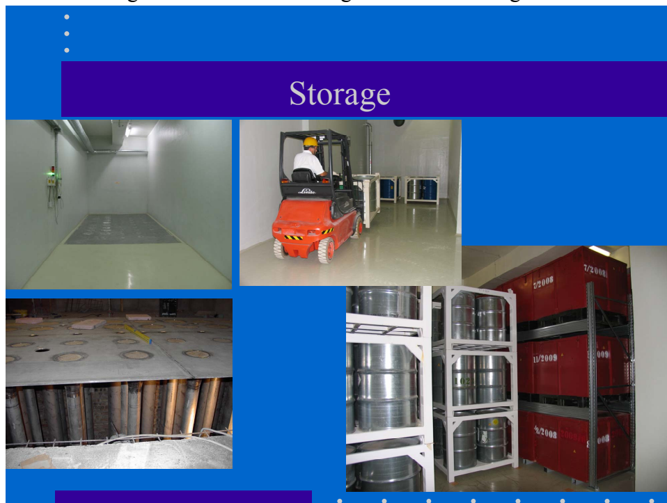
Image 3 – The interim storage rooms and storage wells
