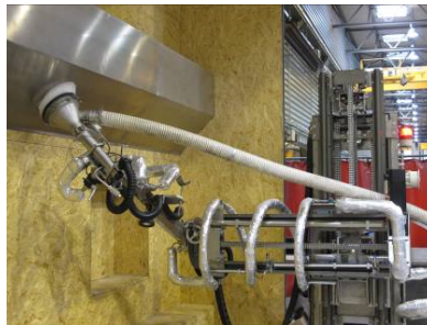
Figure 14 : Test factory acceptance
