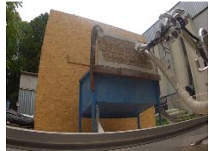
Figure 15 : Test at CTAS-Air Liquide
