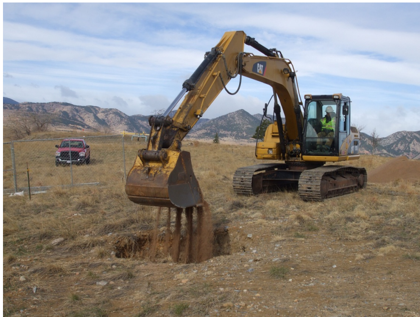
Figure 7. Backfilling the 881 hole in 2011 (excavator provides comparison for the hole size).
