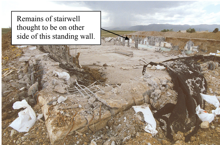
Figure 6. Building 881 after explosive demolition, before backfilling (looking southwest).
