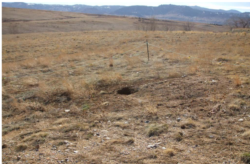
Figure 8. 881 hole approximately 1 year after backfilling.
