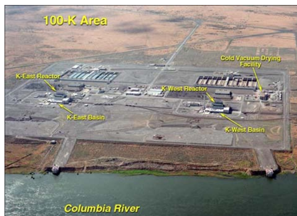
Fig. 1. K East and K West Reactor Basins and the Cold Vacuum Drying Facility.
