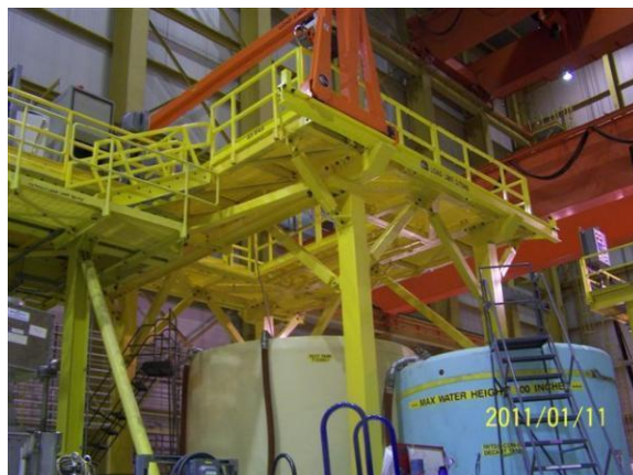
Fig. 2. KOP Full-Scale Test Facility.
