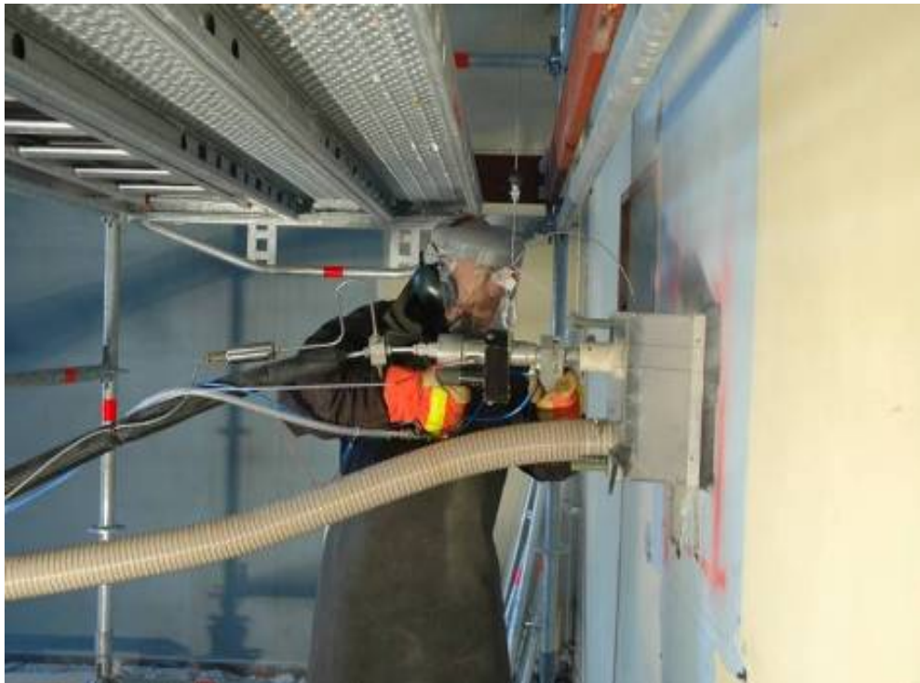
Figure 2: Wall scabbling with Nithrow™
