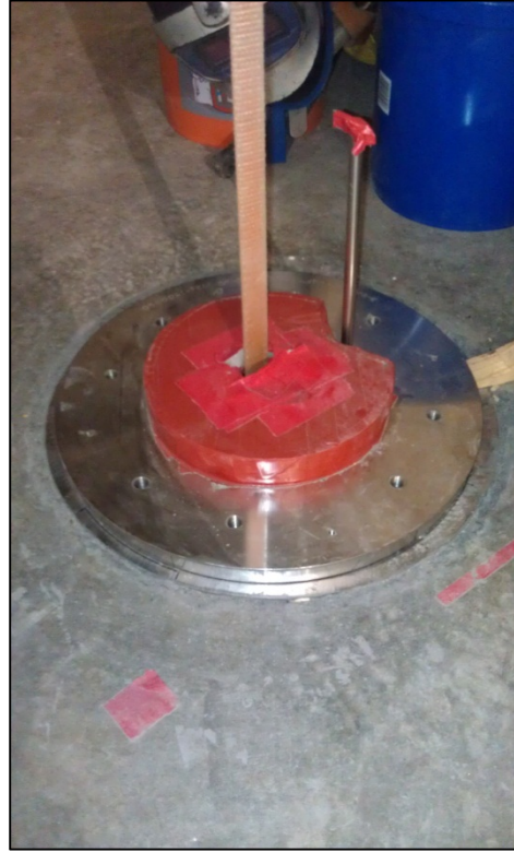
Figure 18: ESV Installation from above the deck
