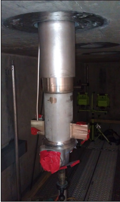
Figure 17: ESV installation from below the deck
