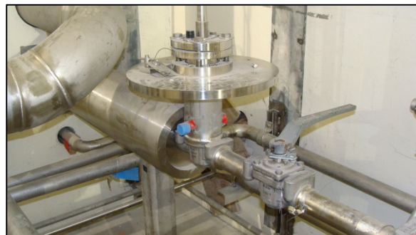
Figure 15: Equipment Installed adjacent to containment
