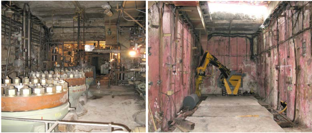
Fig. 4. Use of remote-control mechanisms during equipment dismantlement in room #66.
