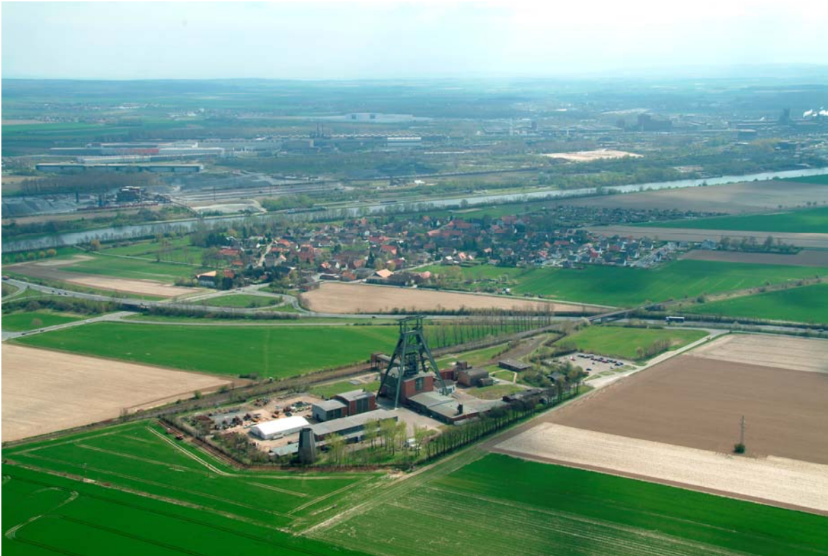
Fig. 1: Aerial view of shaft 1
