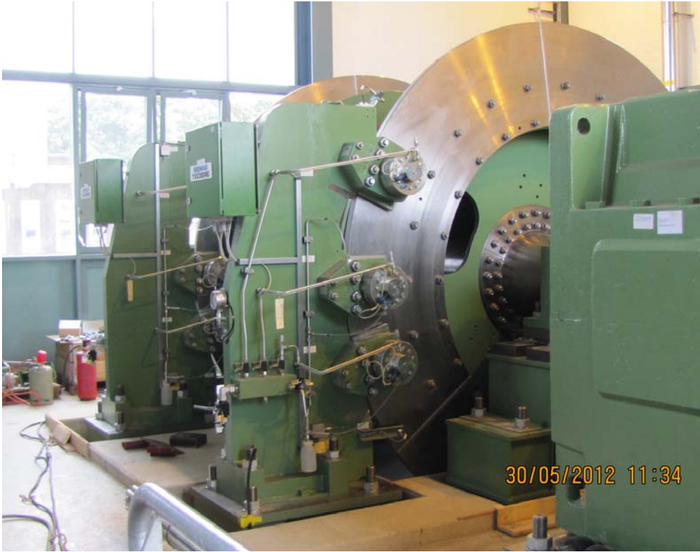
Fig. 5: New hoisting engine Konrad 1 south
