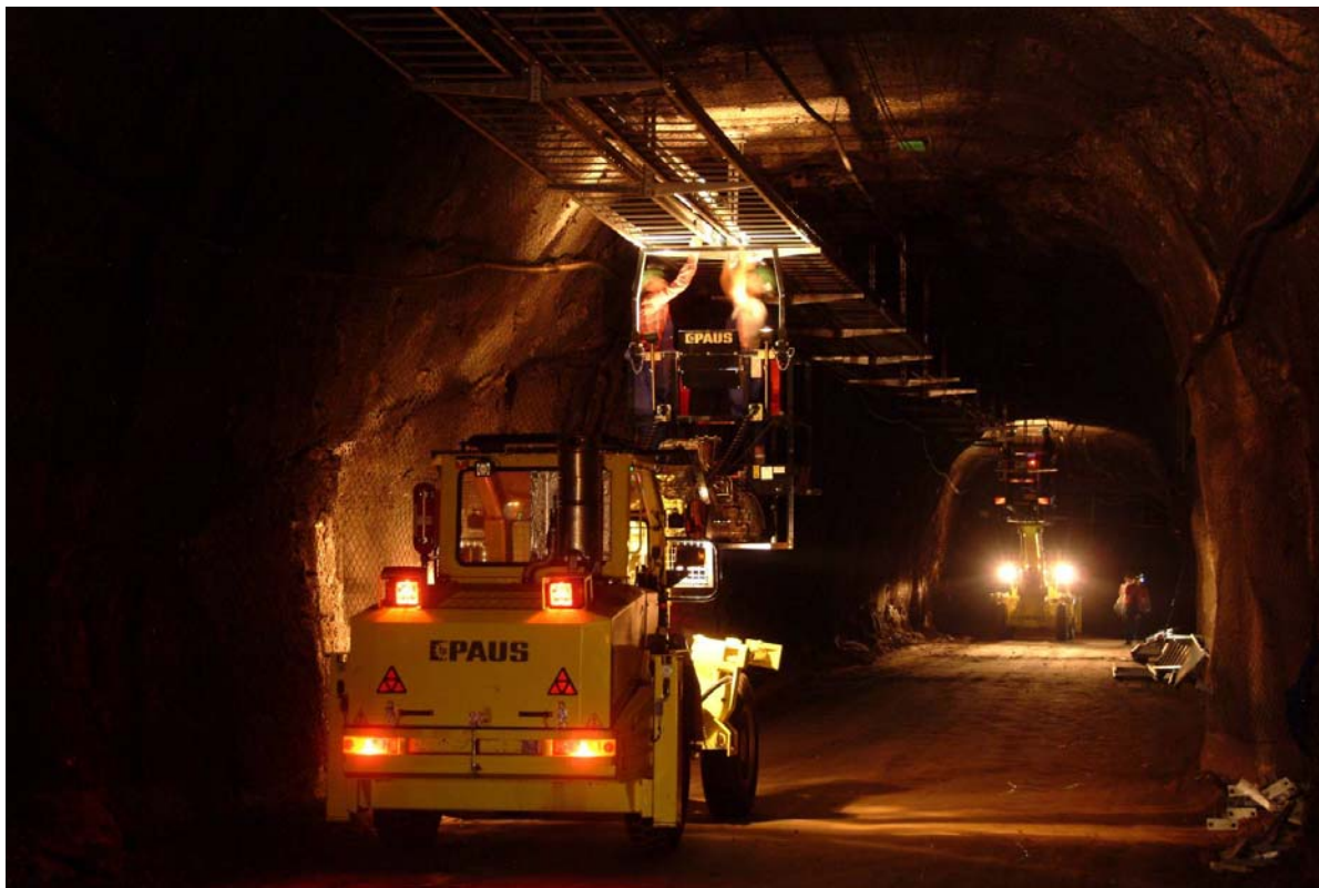
Fig. 6: Underground construction work
