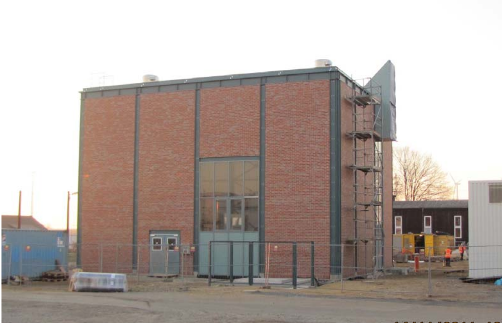
Fig. 4: Hoisting engine building Konrad 1 south
