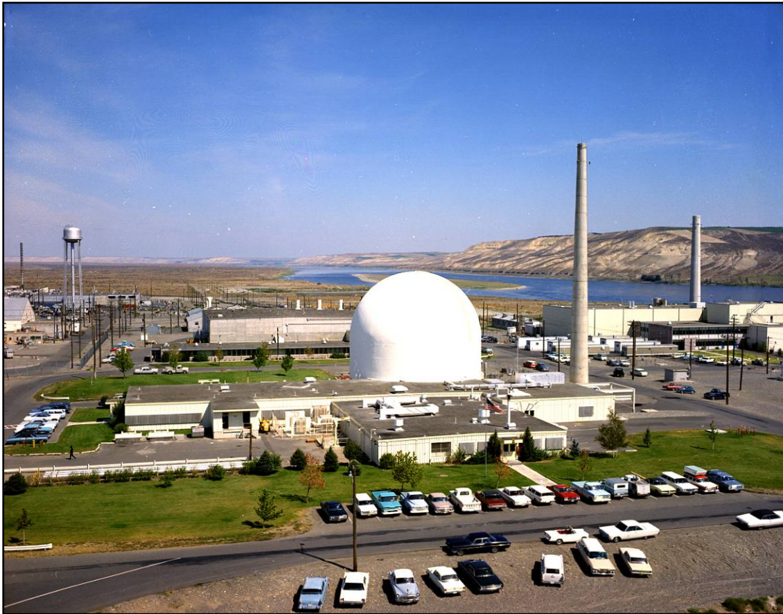
Photograph 1: The 309 Facility in 1968
