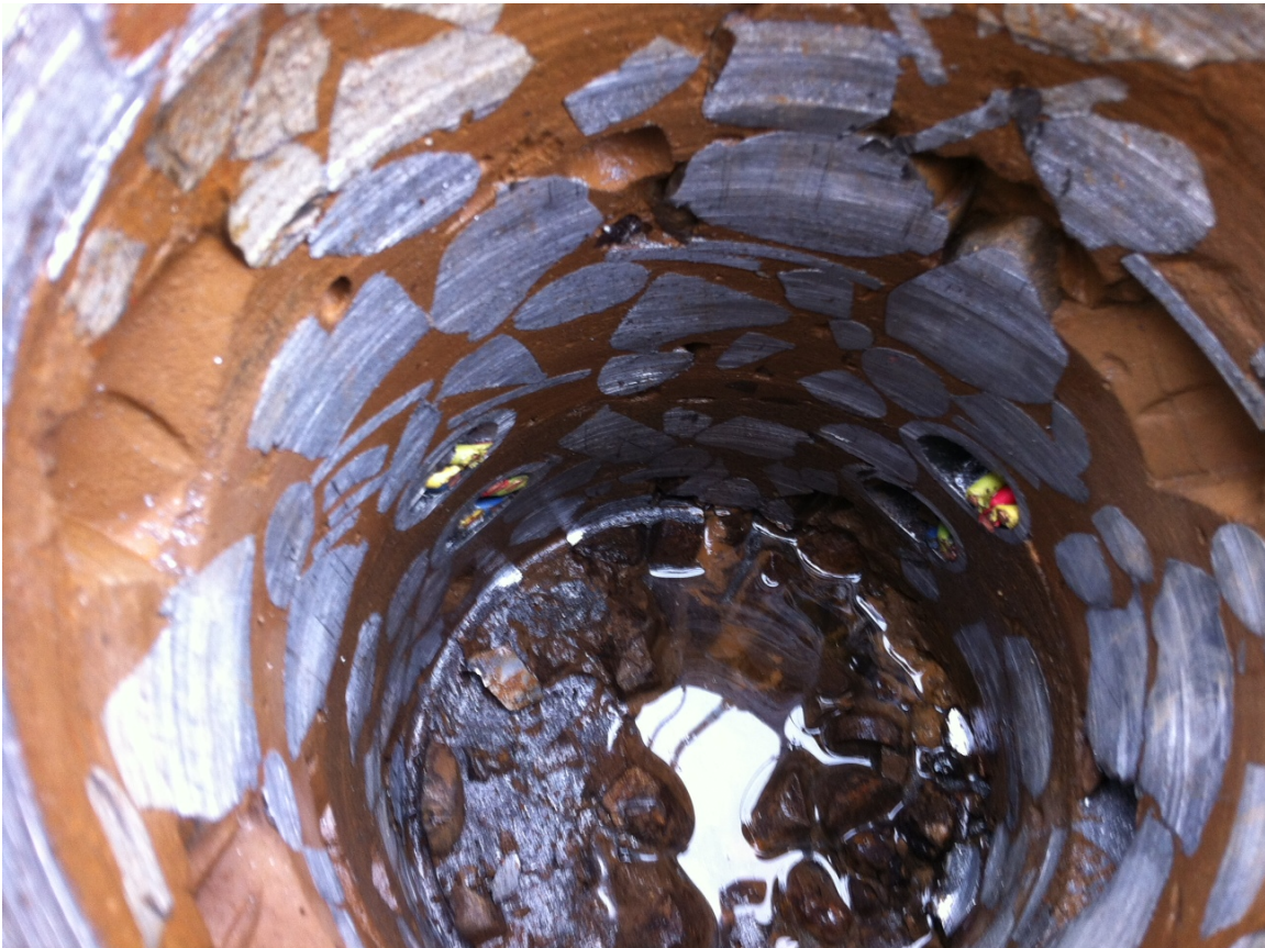
Photograph 2: Thermally Degraded Biological Shield
