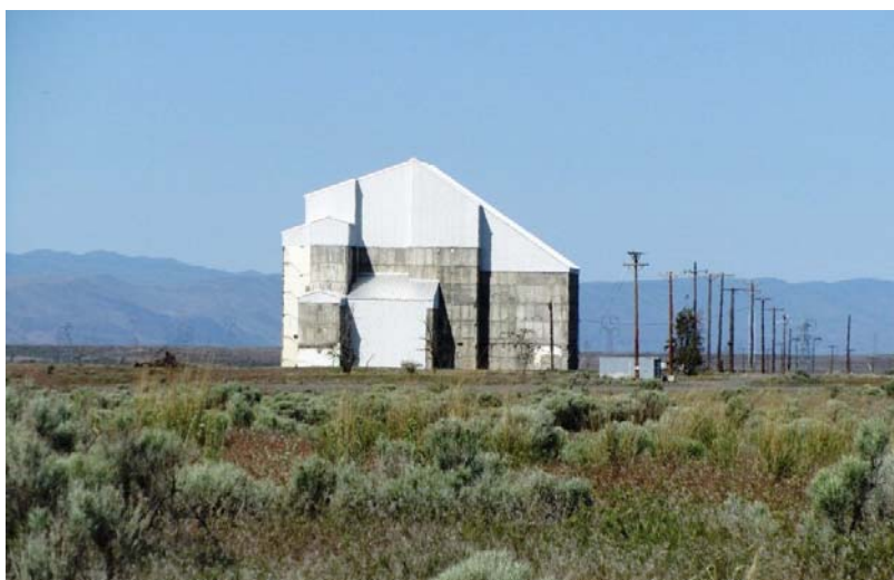
Fig. 2. Cocooned F Area Reactor.
