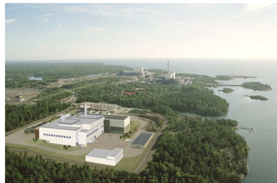
Encapsulation plant in Oskarshamn
