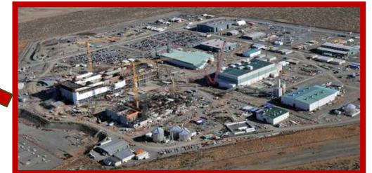
Hanford Waste Treatment Plant (WTP) ($690M)
