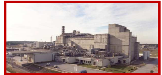
Savannah River Defense Waste Processing Facility (DWPf) ($154M)
