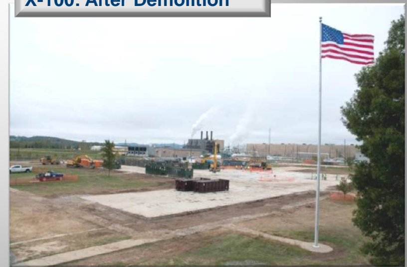
X-100: After Demolition
