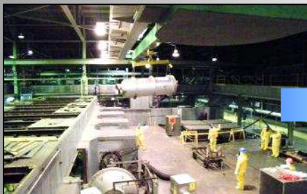
LIFTING TO CART
