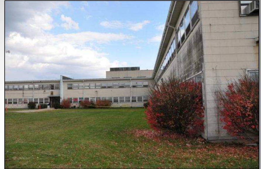
Older X-100 Administration Building
