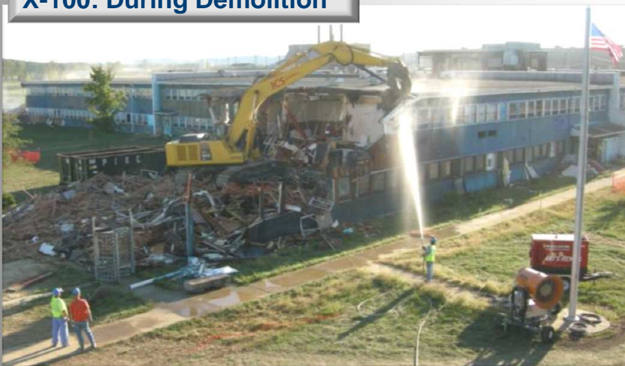
X-100: During Demolition
