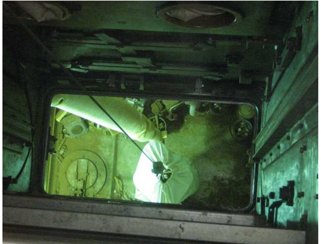
Lifting Waste from Cell 9 into Transfer Case
