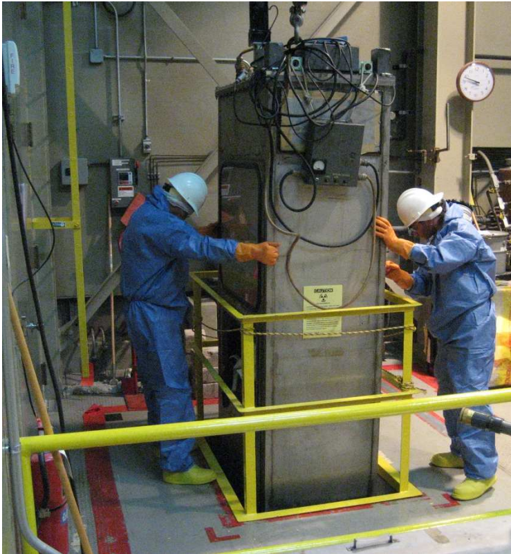
Attaching Transfer Case to Cell 9
