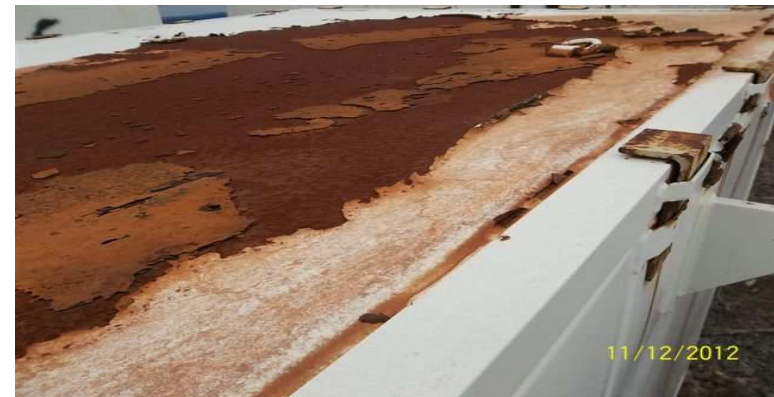
Degrading Top of SP Box on LS 2 Hard Stand
