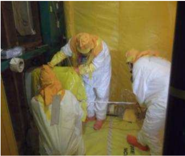
O-14 Building Off-Gas Cell Filter Removal
