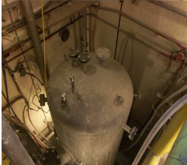
O-14 Building Processing Piping Removal Waste Dispensing Cell
