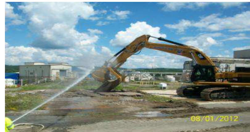
Vitrification Fabrication Shop Slab Demolition
