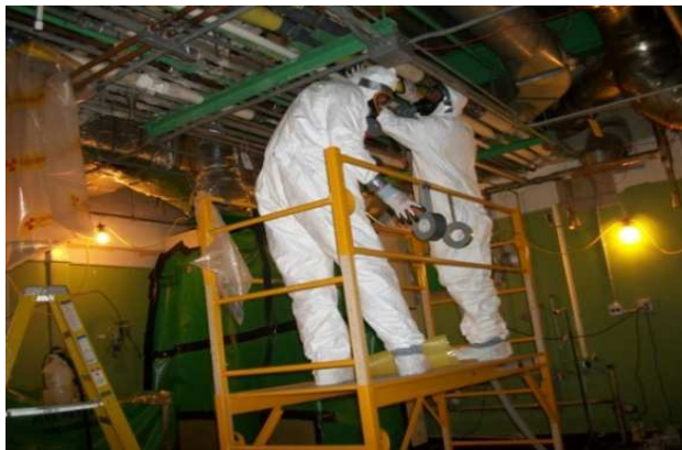
Asbestos Removal Main Plant Processing Building
