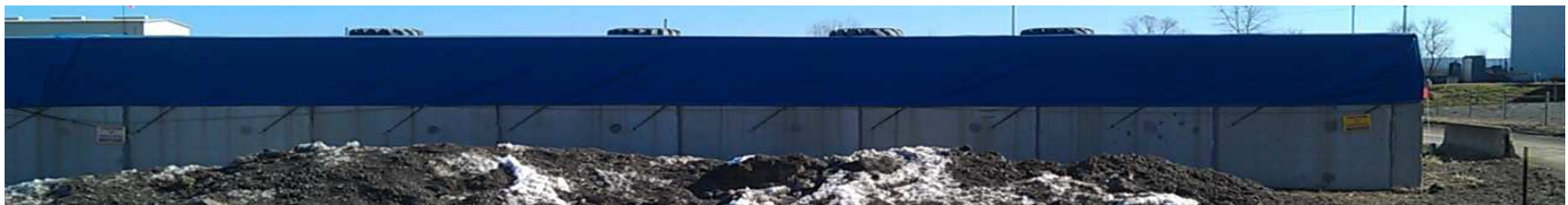
Waste Storage Vaults Containing HLW Tank Pumps and Non-spec Packaging
