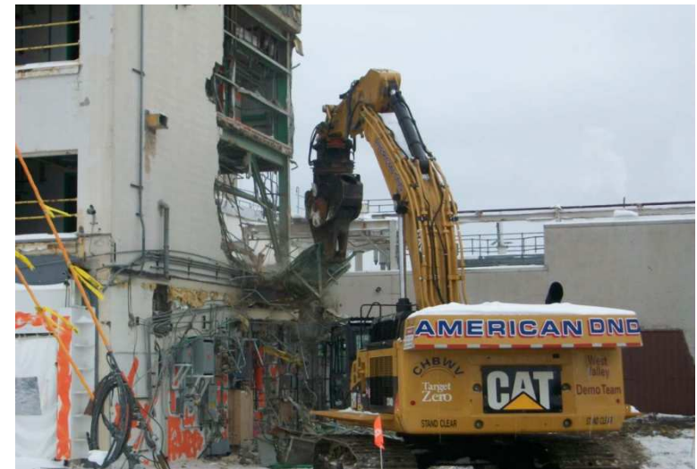
Step 1 Demolition of 0-14 Building
