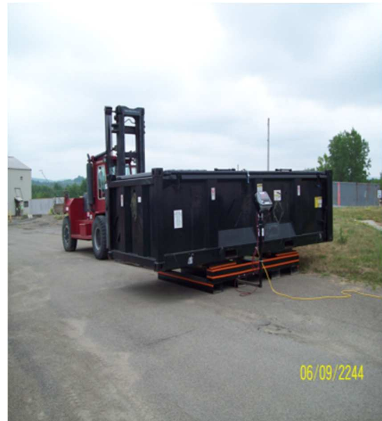
Preparing Intermodals for D&D Activities and Loading of Newly Generated LLW
