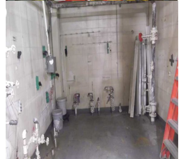
Main Plant Processing Off-Gas Aisle Cleanout
