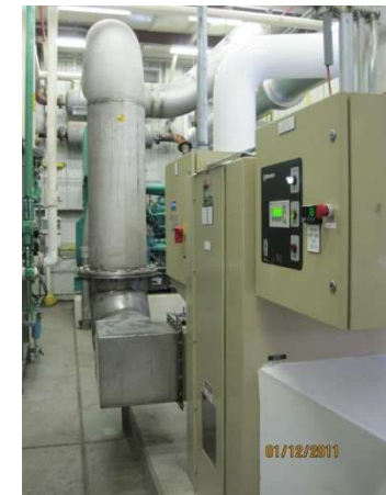
New ventilation ductwork and desiccant drier
