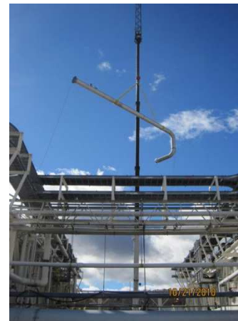
New ventilation ductwork and desiccant drier
